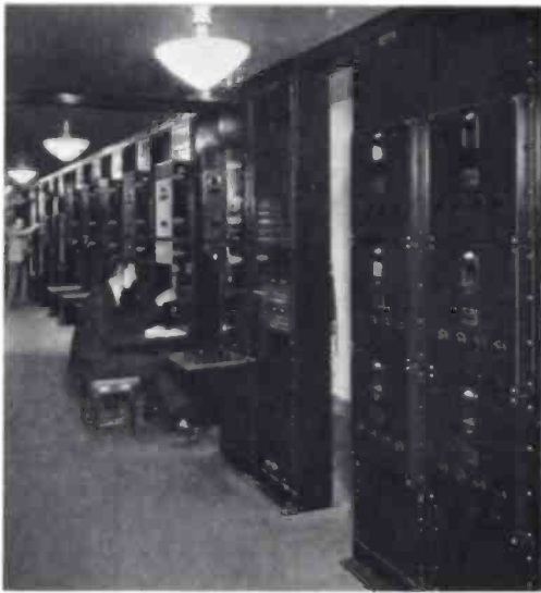
The control room contains twenty-two racks of equipment. The six Western Electric 10-A Radio Receivers are shown on the two racks at the right
