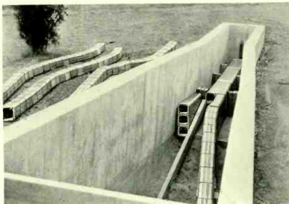
Fig. 7—Concrete-lined trench for studying various types of splays
