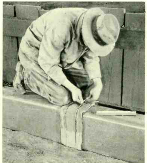
Fig. 6—S. M. Sutton making a mortar-bandage joint in underground conduit
