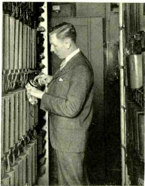
Fig. 2—The dial hand test-set is probably the simplest of all dial test equipment
