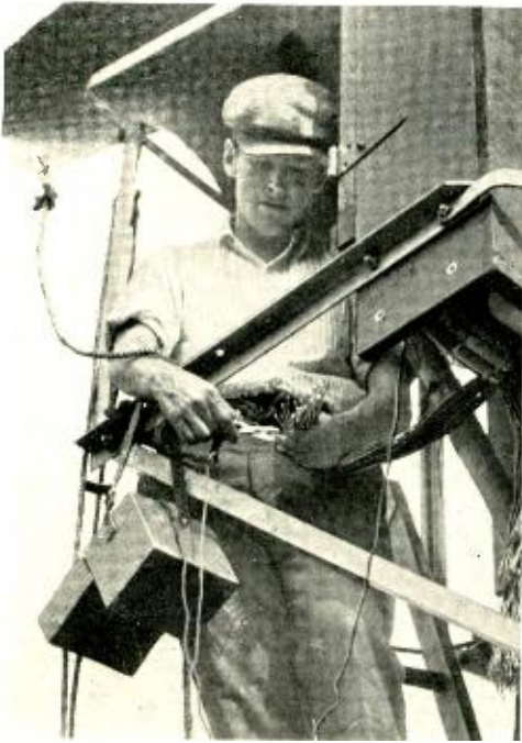
The "receiver-battery" test; contact is made with each wire in turn by the scissors
