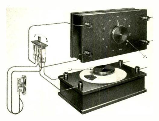
Fig. 1—The attenuators which vary the intensity of tone in the receiver. With the switch in left-hand position, "A" tone is heard; in right-hand, "B" tone is heard
