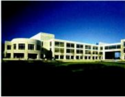
Scientific-Atlanta's headquarters in suburban Atlanta is designed to promote brainstorming among the 1200 engineers who work there
