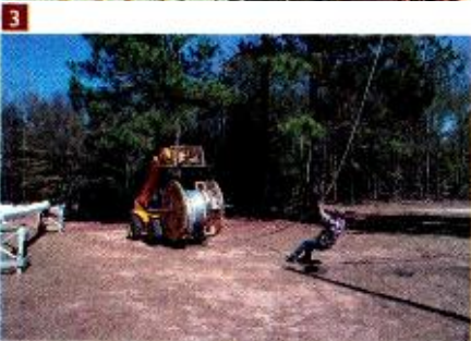
1. Rewiring master control room for digital transmission at WRDW; 2. Channel 31 digital antenna for WRDW; 3. Replacing guy wires; 4. Working aloft on the newly installed digital tower.
