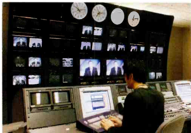
The control room uses a Pinnacle MediaStream 700 server to record programming and interstitials for TV Japan's schedule.
