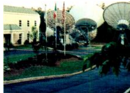
NET/36 operations will be headquartered at PanAmSat's Atlanta facility.
