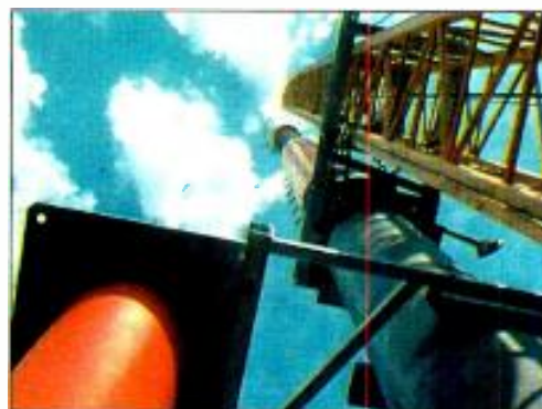
KDFW-DT installs its Andrew TRASAR antenna which is side-mounted with WFAA's new antenna.
