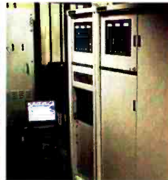
wsb-tv has a new all-digital studio. The station's Harris DTV 100 kw transmitter is outfitted with an ATSC-compliant encoder.
