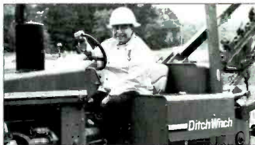
Bob Miron, Advance/Newhouse, atop a trencher in Charlotte, N.C.
