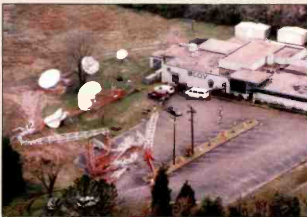
A tornado with winds estimated at 250 mph hit wcov-TV's 800-foot tower 'like a hammer,' snapping it 600 feet up, says owner David Woods.
