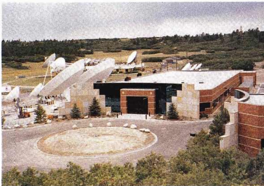
DirecTV control center in Castle Rock, Colo., will provide control of the DBS satellite and will uplink DirecTV programming. Uplink for USSB programming will be in Oakdale, Minn.
