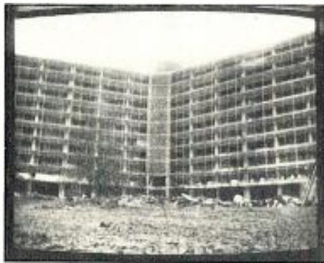
Demolition on KMBC before...
