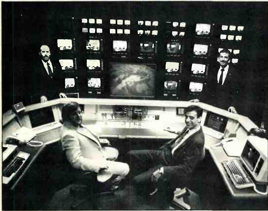
At the controls. NBC's Skypath control room in Burbank is one of two central monitoring facilities of the network's satellite system (the other is in New York), and is used to direct switching information for the 160-plus affiliates using Ku-band satellite earth stations. Above, seated, are on-air technical managers Pat Walsh (l) and Michael Harabin (r), and standing are Steve Orland, director, on-air operations (l), and Mike DiPalma, manager, satellite operations (r).
