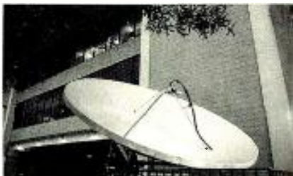
The Florida Network's permanent uplink in Orlando distributes programming via two SCPC carriers on Westar III.
