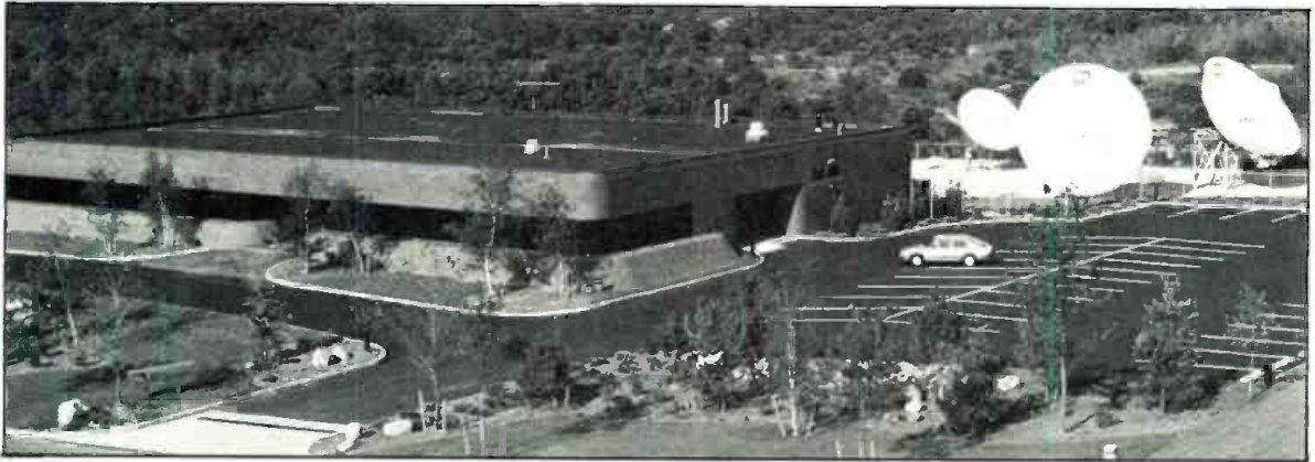
WA's network operations center on Long Island
