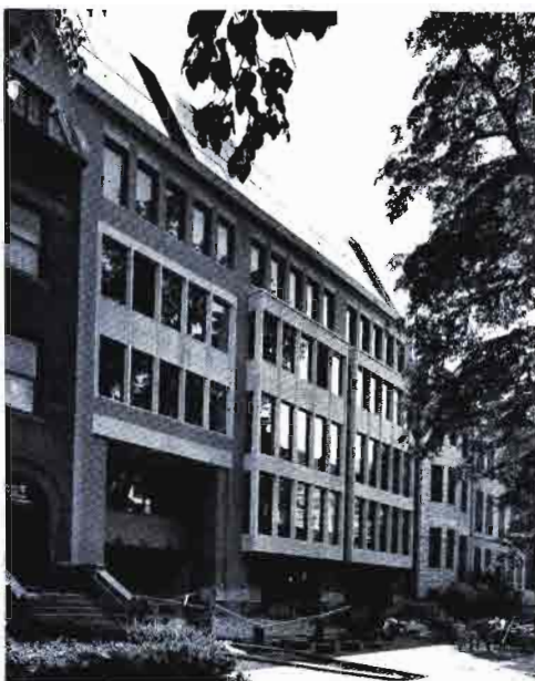
NCTA $750,000. Some space in the 40,000-square-foot structure will be made available for sublease to lawyers or nonprofit organizations that fit the area's "special purpose" zoning. The prestigious street includes the embassies of Canada and Chile, and the headquarters of the Brookings Institution.
