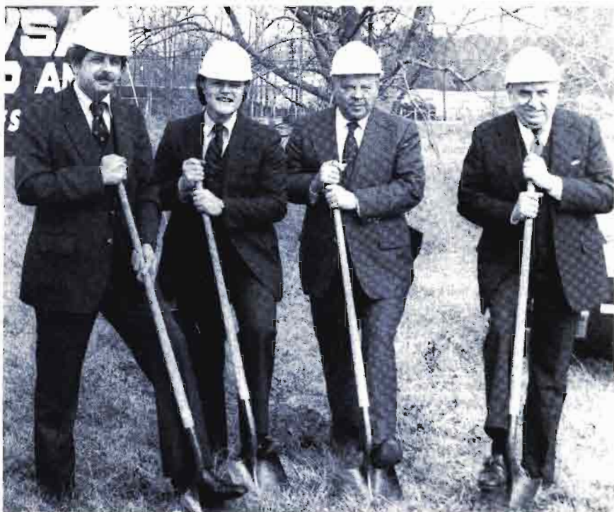
Getting in their digs. Groundbreaking ceremonies for the new facilities of WWSA(IAM)-WCHY(FM) Savannah, Ga., were held March 12. Located on Alford Road in the western part of the city, the structure will cost more than $250,000. Welding the shovels were (l-r): William Sanders, executive vice president, Georgia Association of Broadcasters; Truman W. Conley, vice president/general manager of wwsa-wchy; Vincent T. Wasilewski, National Association of Broadcasters president, and H. Hart Hogan, president of Bluegrass Broadcasting Co., which bought the stations last summer.
