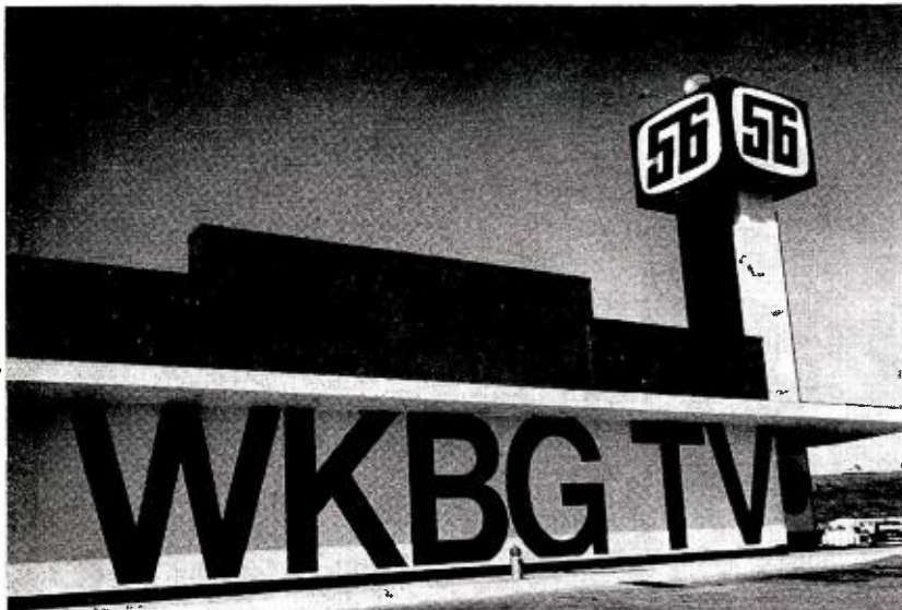
WKBG-TV Cambridge-Boston has completed construction of a $2.5-million facility that houses two large color studios and spans 44,000 square feet of space. The new plant is at 75 Morrissey Boulevard, adjacent to the Southeast
