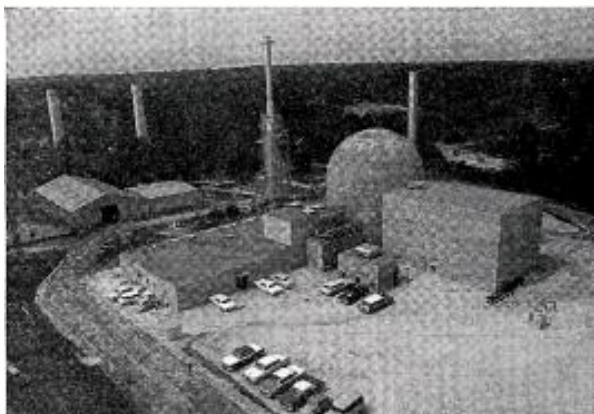
Atomic Plant, Parr, S.C., built for Carolinas Virginia Nuclear Power Associates.
