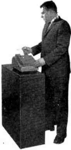
AUTOMATIC PROGRAM LOGGING . . . New ATC development that automatically prints FCC logging information directly from magnetic tape as it is broadcast.
