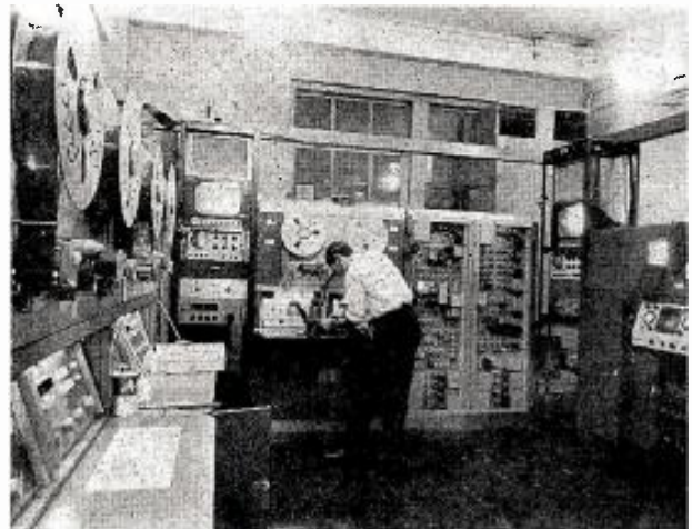
Complete tape facilities for playback, editing and recording are contained in this new tape control center at New York headquarters.
