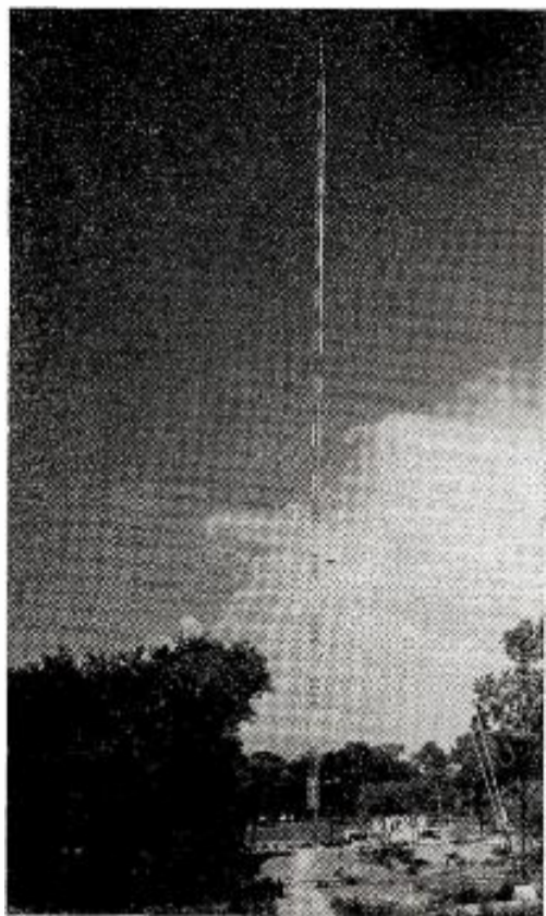
Higher than ever • KTVI (TV) St. Louis, whose 592-ft. tower was toppled by a tornado last winter (BROADCASTING, Feb. 16), now is operating from a new 1,049-ft. Kimco tower. At the base is KTVI's new 100 kw transmitter. The new gear cost about a half-million dollars.
