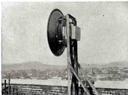
Microwave reflector with transmitter on back, at Roanoke, Virginia.
