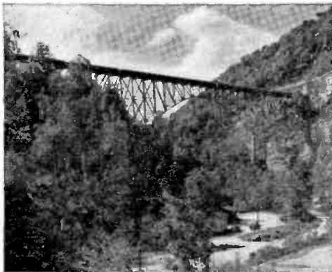
Bridge-Builders Paradise is the recently completed West Virginia Turnpike. Its 88-mile length required 76 bridges, built from 23,500 tons of steel. The Bender Bridge, here, is 278 feet high, one of the tallest bridges east of the Mississippi. U. S. Steel supplied the steel and built this bridge.
