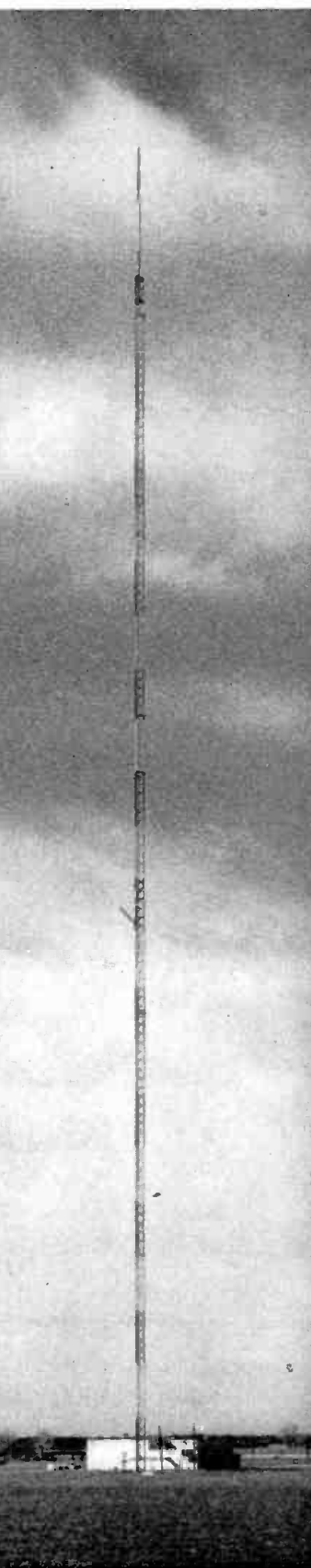
EMSCO guyed TV Tower over 1000 ft. in height, Great Bend, Kansas
