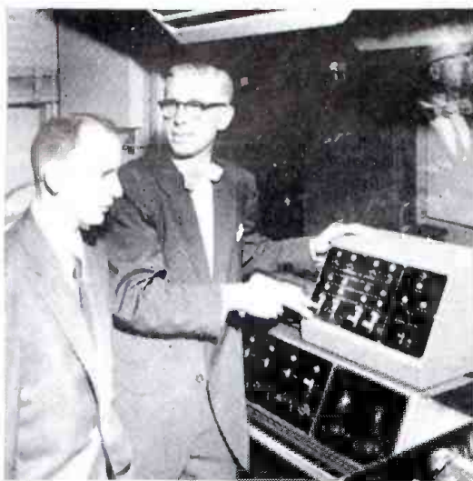
ERNEST DEUTSCH (l), broadcast engineer for Standard Electronics, and Ralph Schlegel, technical facilities supervisor for WOR-AM-FM New York, watch the Studicon control box in operation in the control room of the station. Mr. Deutsch designed and developed the Studicon unit.
