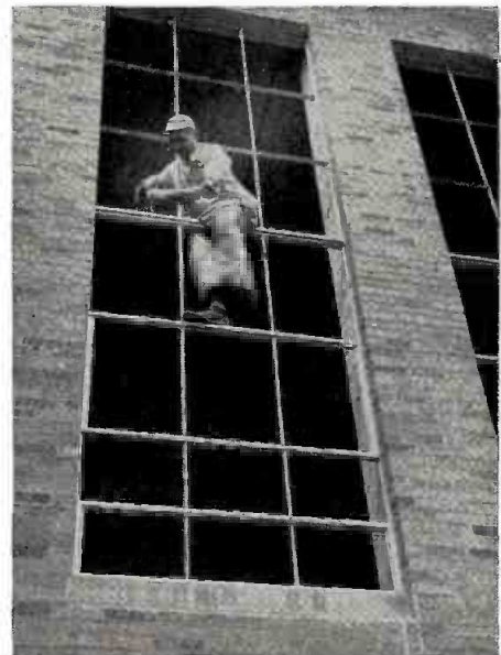
A Quarter Ton Of Glass must be supported by the sash in this convent-school. The sash is double glazed with stained glass on one side, clear glass on the other. Because of the great weight, and the high winds in the area, the authorities chose steel windows because they are so strong. For many years, United States Steel has furnished special rolled steel window sections for manufacturers all over the country.
