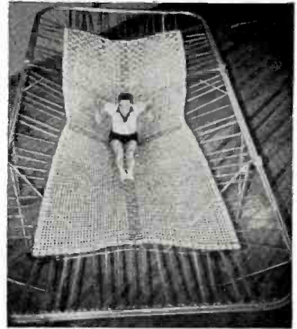
The Spring's The Thing that gives a Trampoline its unique place in the world of exercise and entertainment. Around the edge of the resilient "bouncing" surface, more than 100 oil-tempered springs, carefully designed and precisely manufactured by U.S. Steel, quietly go about their jobs of supplying the "motive" power that enables a performer to bounce and leap as high as 26 feet.
