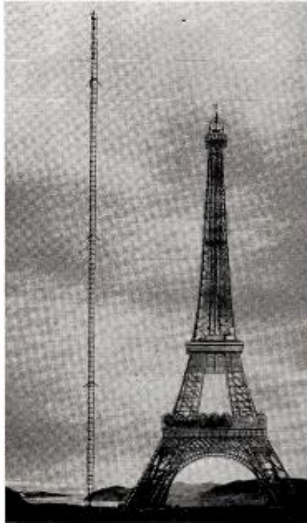
THIS MONTAGE compares Truscon's 1,218-foot tower at Thule AFB, Greenland, with the 985-foot Eiffel Tower, granddaddy of all giant steel towers.
