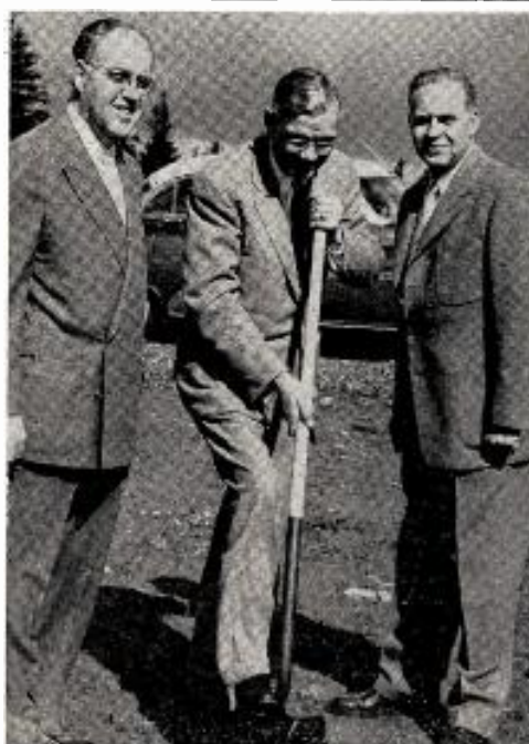
OREGON Gov. Paul Patterson (c) breaks ground for KOIN-TV Portland's new 708-foot, $135,000 tv tower, expected to be complete July 1 when power will be increased from 56 to 100 kw. Flanking the governor are C. Howard Lane (l), station's managing director, and Louis S. Bookwalter, engineering director.
