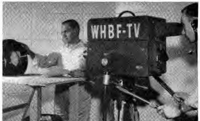
Here's how WHBF-TV puts UP facsimile newspaper pictures on the air. Pictures are mounted on old transcriptions like one held by Bob King (l), engineer. Tv camera, operated here by Earl Hill, is set so facsimile fills screen.
