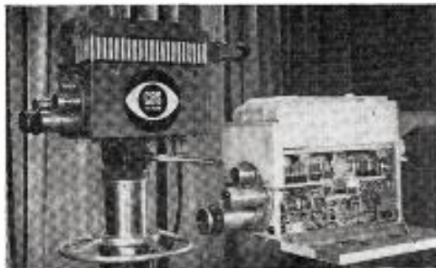
COLOR camera at right is comparable in size to the standard black-and-white tv camera shown at left. The color tv camera is the new Chromacoder developed by CBS Labs Division and basically reflects further refinement of the field sequential camera which has been in operation since 1946. It contains one orthicon image tube and is portable for remote pick ups.
