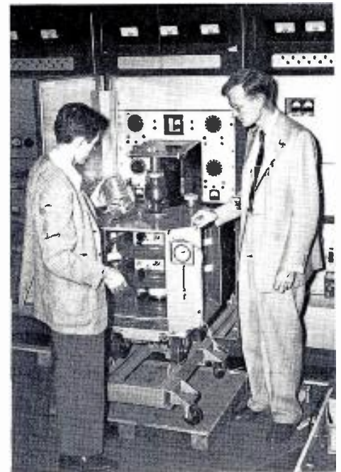
DON WILLOUGHBY (r) Chief Engineer for Television Station WNOK-TV, Columbia, S.C., inspects the roll-out dolly which houses the tuning coils and the Eimac klystron amplifier for the high powered Du Mont 5 KW UHF television transmitter delivered to WNOK-TV. Stan Pauloski, Research Engineer for the Allen B. Du Mont Laboratories, Inc., is explaining the operation of the unique, easily accessible dolly during last checks prior to shipment of the transmitter.
