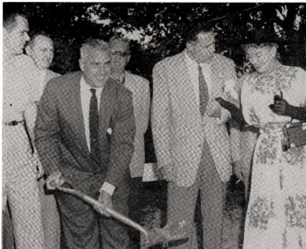
SILVER SHOVEL was used in groundbreaking ceremonies for WRTV (TV) Asbury Park, N. J. Wielding shovel is F. Bliss Price, mayor of Eatontown, the town in which the WRTV transmitter will be located. He is flanked (l to r) by Jackie Cooper, TV, stage and screen actor; Paul Peterson, assistant general manager for Walter Reade Theatres; Hervey Keator, manager of the Eatontown Drive-In, where the studio and tower will be located; Walter Reade Jr., president of the theatre organization and WRTV, and Hildegard, the songstress. The groundbreaking ceremonies were held Aug. 15. Mr. Reade said the station, on uhf Ch. 58, will program features of local interest which cannot be obtained from New York outlets. Commercial programming is set for late December.
