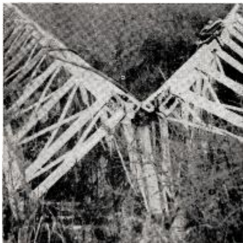
FOUR twisted pieces were all that remained of one of the towers of WGAI Elizabeth City, N. J., after the Aug. 13-14 hurricane struck.
