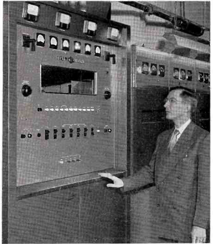
G. Edward Hamilton, Eastern Division Television Engineer for ABC, inspects the aural cubicle of a new General Electric 20-KW Amplifier.
