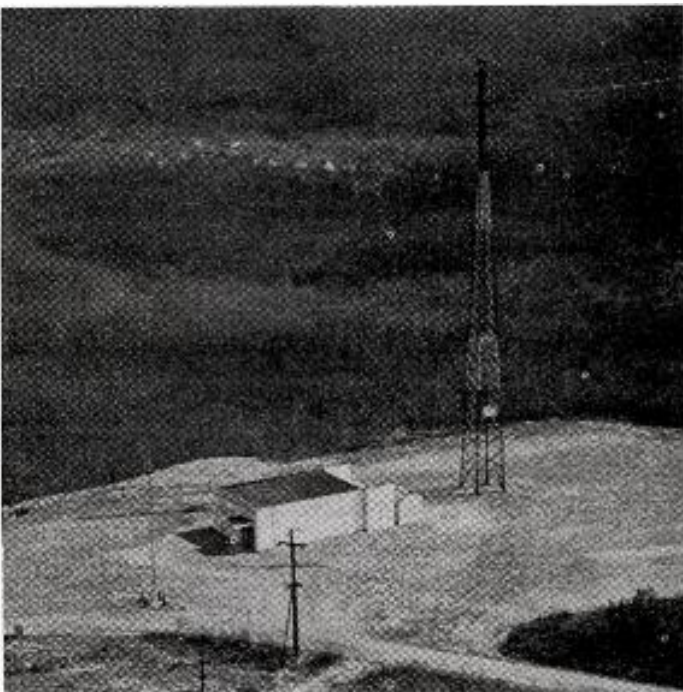
WFBG-TV's new General Electric 12-Bay Antenna was erected atop Mt. Wopsy, overlooking the beautiful Pennsylvania terrain.
