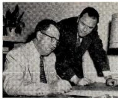
WICC-TV President Merryman (l) signs contract with Thomas Gallatin of Graybar Electric Co., which will furnish uhf equipment for station.
