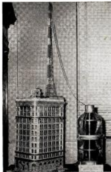
SCALE model of proposed TV tower and antenna installation of WSAV-TV Savannah, atop bank building. At right is a 300-millimeter Aviation Obstruction Electric Code Beacon, which would be installed atop the tower. WSAV's TV application is now pending before the FCC.
