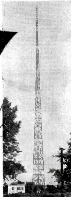
Truscon Self-Supporting Tower, operated by WEMP-FM, Milwaukee, Wisconsin, is 410 feet high with Western Electric 6 Unit Cloverleaf FM antenna.
