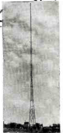
This 240 foot Truscon Tower, operated by WTCH, Shawano, Wisconsin, has 52x48 Truscon Ground Screen to assure an excellent signal.
