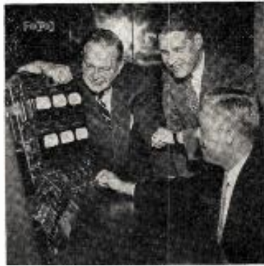
FLICK of a switch by Chris J. Witting (r), director and general manager of DuMont TV Network, launches operation of WABD (TV) New York transmitter from atop the Empire State Bldg. in New York. Signal is given by Rodney D. Chipp (c), network director of engineering, while Clarence G. Alexander, DuMont operations director, looks on. Station's transmitter went on the air from new site Oct. 26.
