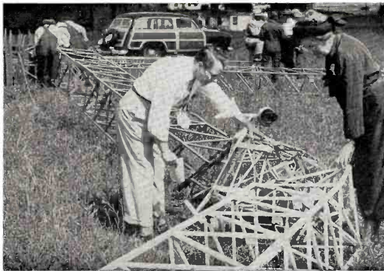
A SUDDEN windstorm snapped guy wires, twisted and toppled one of the 300-ft. antennas belonging to WVOK Birmingham, Ala. Alert engineers cut power flowing to the fallen antenna and station continued operation without loss of a minute of air time. WVOK also was able to warn Birmingham residents of the storm. Examining the twisted framework are (in foreground) Ire Leslie, WVOK program director, and Mrs. Iratee W. Bennis, WVOK president.
