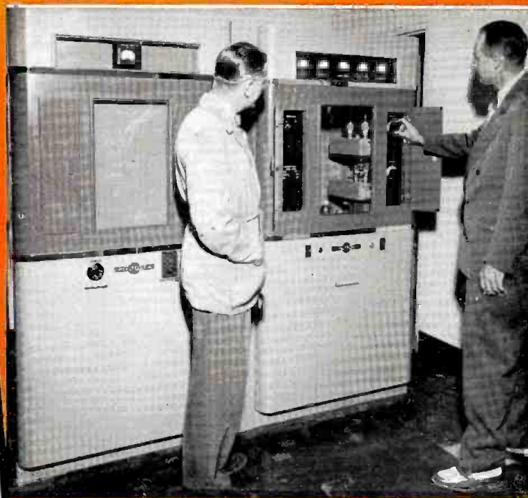
Maxwell Kelch, owner and General Manager of the Nevada Broadcasting Company, at the controls of the new Collins 20V one-kilowatt AM transmitter. At his left, J. E. Tapp, head of T & T Radio Measurements Company and KENO's Consulting Engineer. Back of Mr. Tapp is the phasing equipment in matching cabinet.
