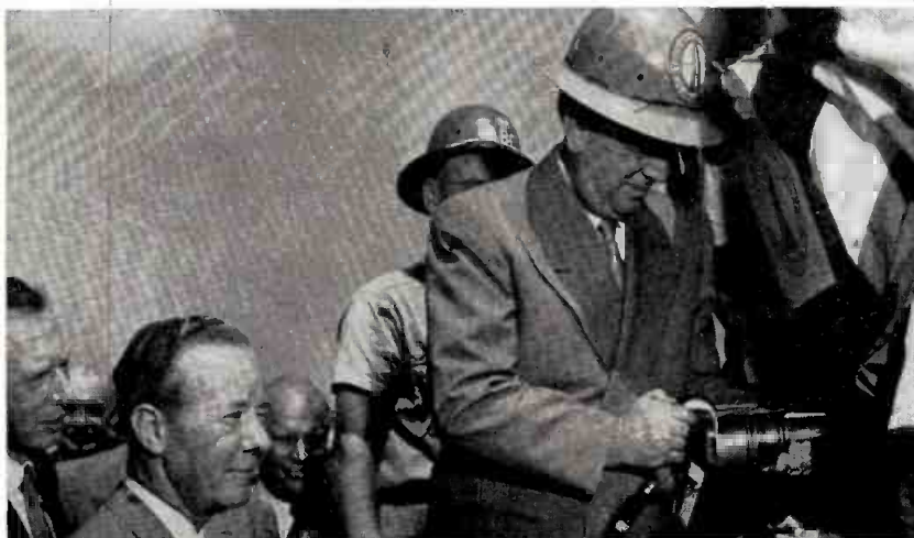
CEREMONY starting construction of the new 217-ft. TV antenna atop New York's Empire State Bldg. finds Mayor O'Dwyer hammering in a gold-plated rivet. Watching are (l to r) Lawrence W. Lowman, CBS vice president; Mark Woods, ABC vice chairman; Dr. Allen B. DuMont (in background), president, DuMont Labs.
