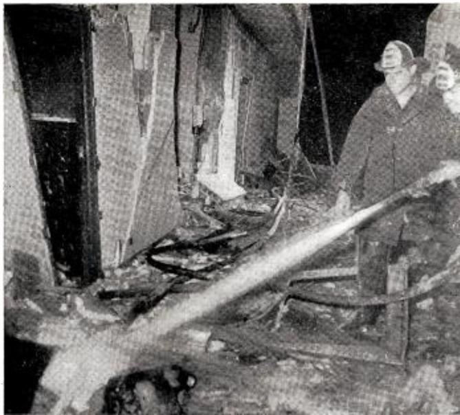
FIREMEN wet down ruins of 8th floor corridor near FCC docket room after fire is brought under control. Major explosions of transformers and other electrical equipment occurred in this area.
