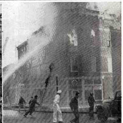
top floor. Station returned to air that afternoon with a broadcast of the Purdue-Illinois game using two old studios in a portion of the building not as badly damaged and new equipment rushed from Gates Radio Corp. manufacturing plant in Quincy, Ill.
