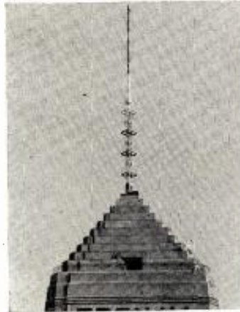
Uppermost portion of Minneapolis' famed Foshay Tower and multi-purpose antenna.
