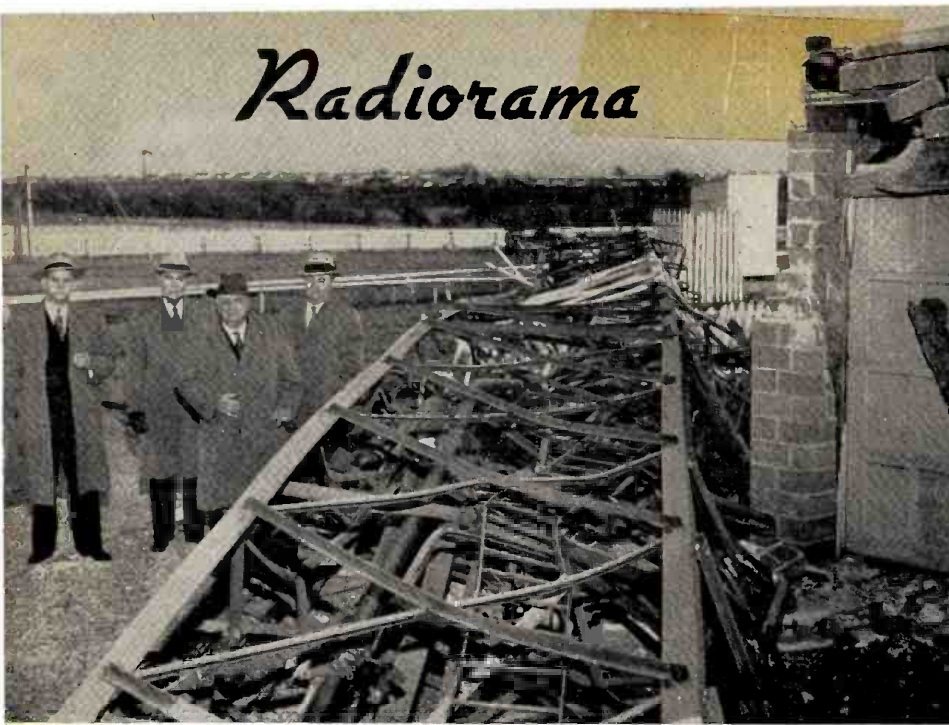
INSPECTING wreckage of the KRLD Dallas towers, located near Garland, following their collapse Dec. 21 (see story this issue) are (l to r) Clyde Rembert, manager of KRLD; Don Houseman, insurance executive; Tom C. Gooch, president of The Times-Herald , station owner, and John W. Runyon, KRLD president. Station resumed in about eight hours.
