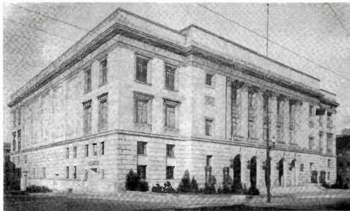
FOUR-STORY MARBLE structure owned by the American Red Cross in downtown Kansas City, Mo., soon will become the new home of KMBC and KMBC-FM.
