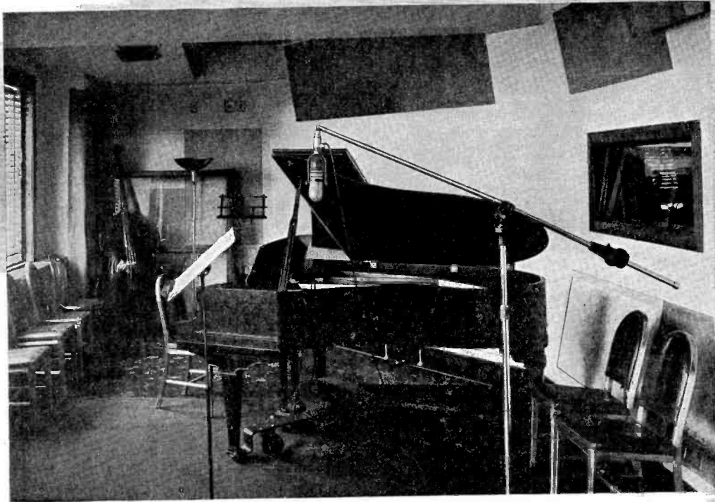
Studio of FM Station WLOU, Detroit, Michigan. RCA 77-B Microphones are used in this studio and RCA 88-A Microphones in the announce booth.
